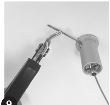
Cut the Suspension Wire to the desired Wire length.
